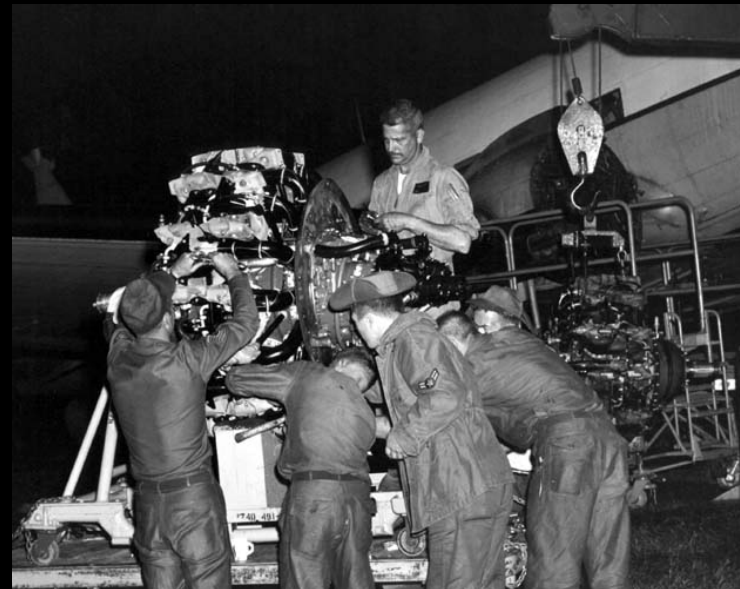
7th ACS Flight Engineer and Maintenance work on a C-47 engine.
